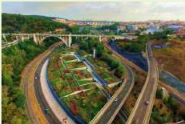
Green roof of WWTP in Alcântara (AdTA, 2018)
