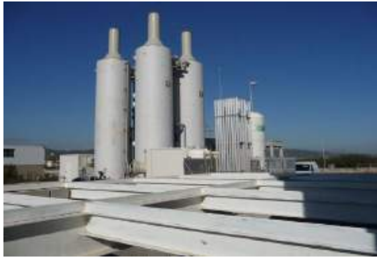
Figure 63: Stripping towers in Estrella wells.
