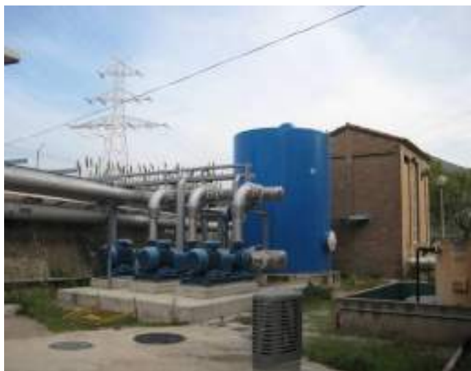
Figure 59: Abstraction pumping groups of Besòs DWTP.
