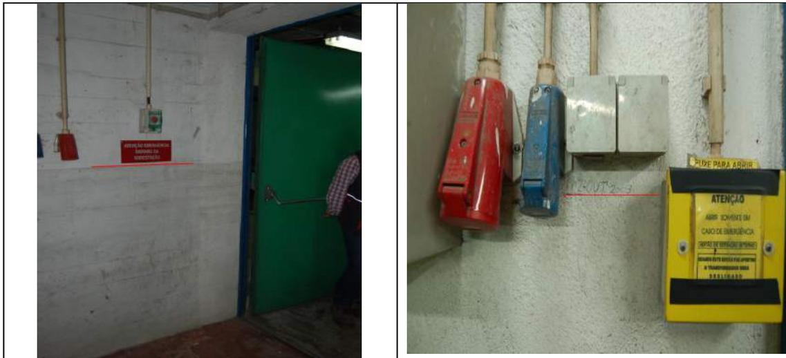
**Figure 76: Flood level registered in the walls of the flooded substation.**
