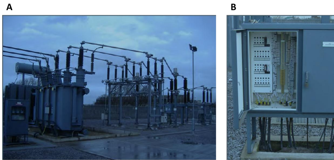
Figure 8: (A) 132kV Grid substation with main power conductor at high level and control circuits located in cubicles at lower level, (B) Cubicle at low level susceptible to flooding (Energy Networks Association (2009)).
